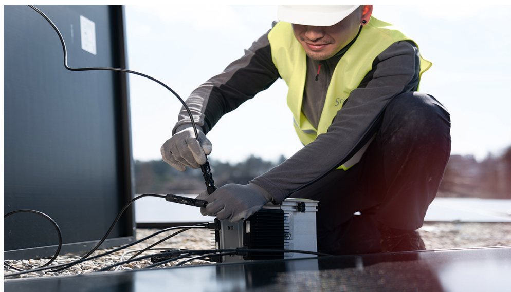
Avoid cross-mating of PV connectors from different manufacturers and only couple same brand connectors
