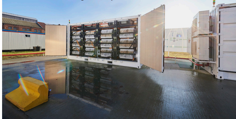
Connected Energy's 1.2MW/720kWh BESS project assembled using Renault second-life EV batteries at an industrial site in Belgium, Europe.
