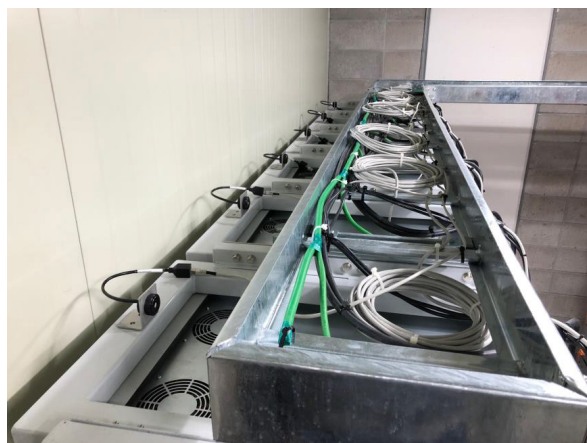
Smoke and off-gas detection monitoring sensors, mounted on top of lithium-ion battery racks.
