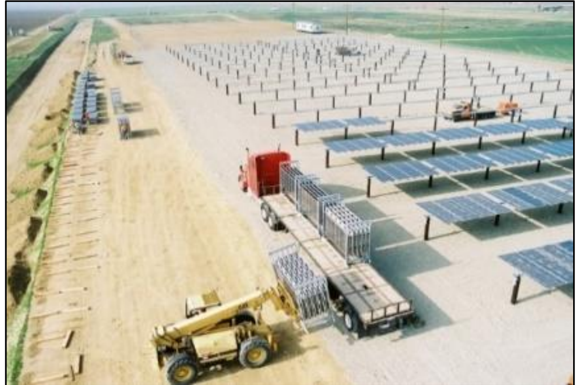
2004; 1 MW, Pre-Panelized "Panels" consisting of 2 CEE purlins & 6 Shell Solar PV modules of 0.55m width for a 3.3m chord
