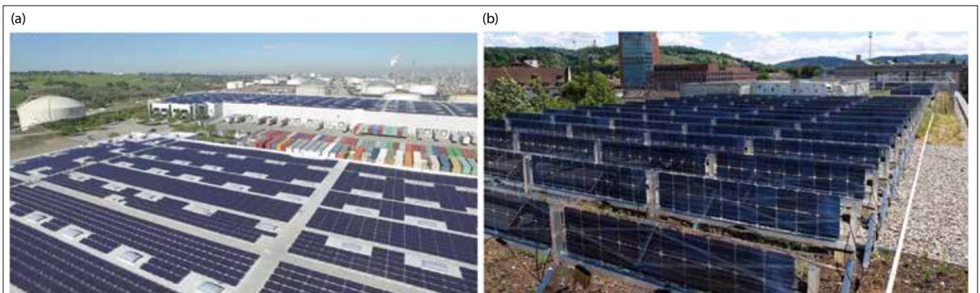
**Figure 4. (a) 10 MWp bifacial fixed tilt installation by sunpreme (USA) [42] and (b) bifacial vertical installation by Solarspar (Switzerland) [43]**
